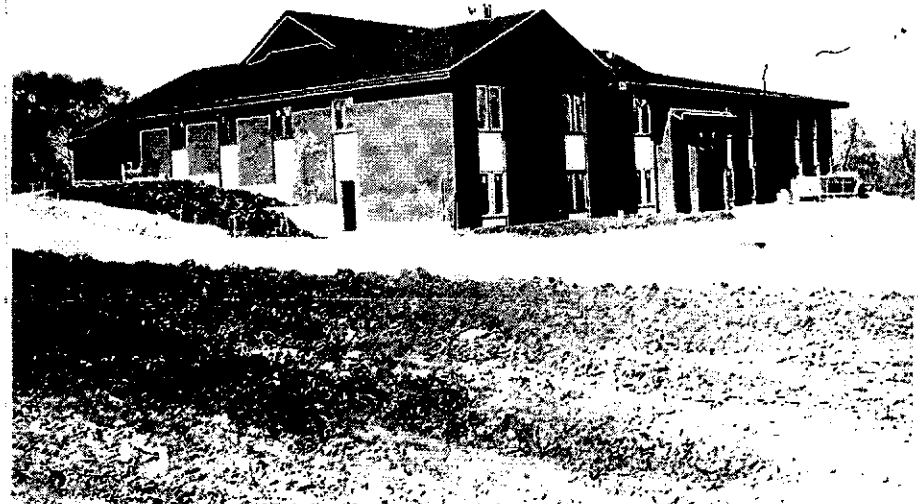
The top photo shows the new municipal building as it appears from Bloomingdale Road. The picture above, which was taken from the southeast, reveals the lower level and the parking lot.
