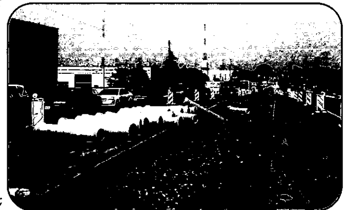
Rows of sewer pipe awaiting installation
