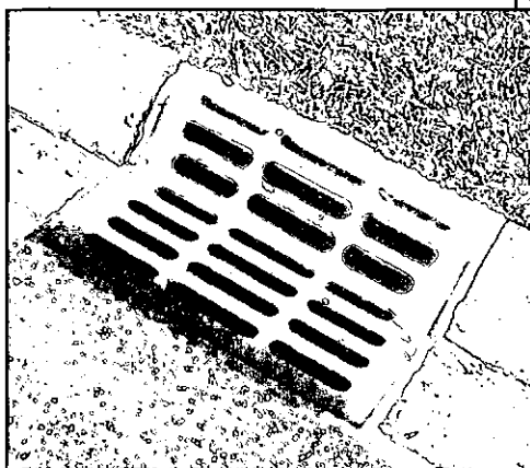
Storm inlet cleared of debris
